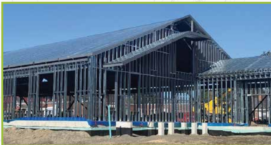
Northern Light CA Dean new hospital construction.
